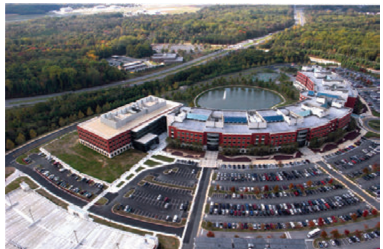
The Defense Threat Reduction Center at the McNamara Headquarters Complex, Fort Belvoir, Virginia
