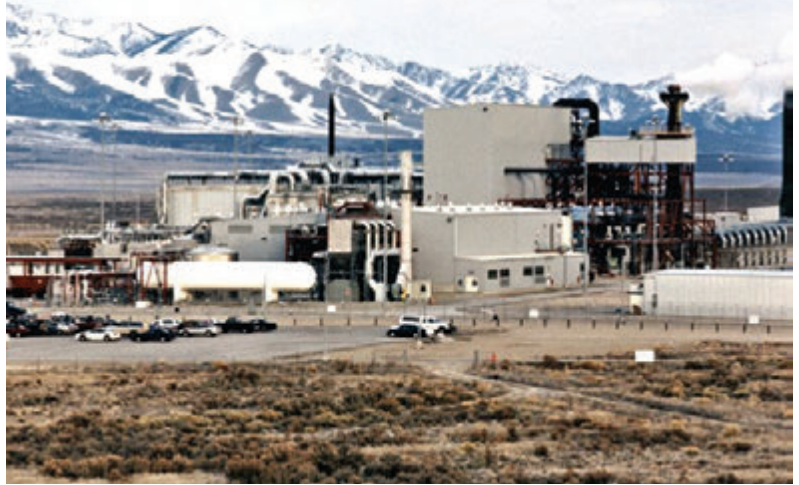
Chemical Demilitarization Plant at Tooele, Utah
