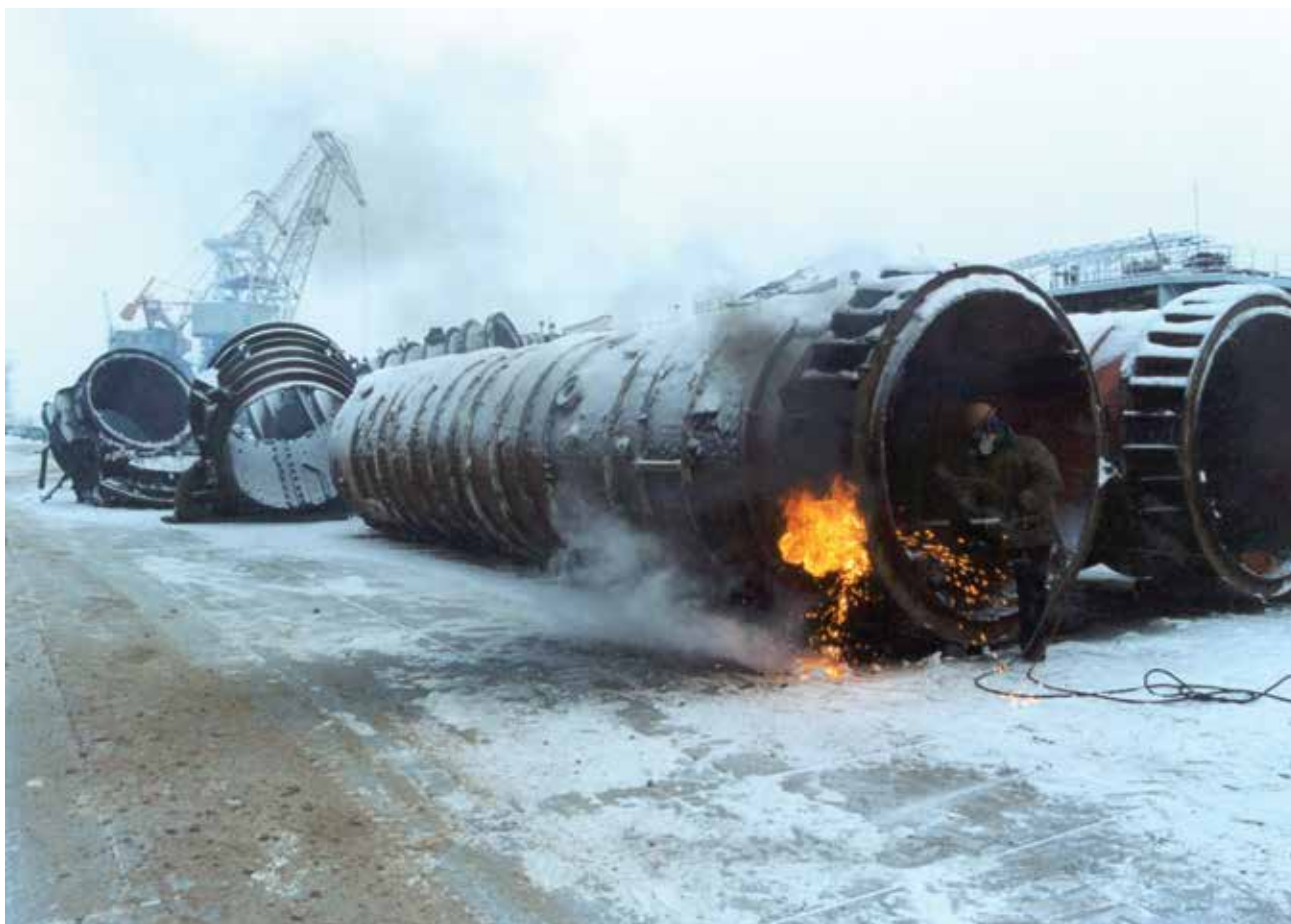
Elimination of SLBM launch tubes
