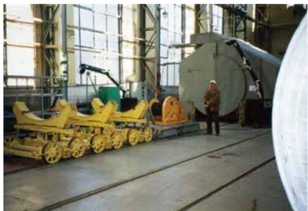
Inside CTR renovated warehouse at Dnepropetrovsk, 1998
