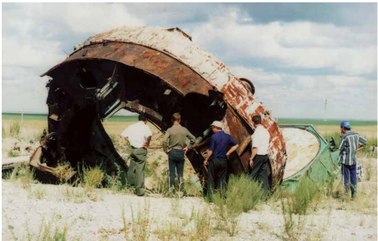
Ukrainian workers at SS-19 launcher silo complex
