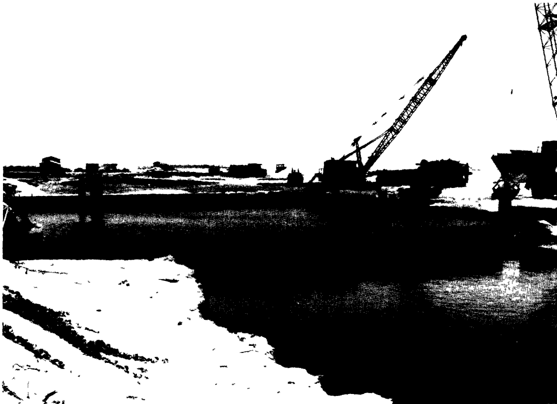
FIGURE 6-15. AOMON CRYPT JUST BEFORE BACKFILLING. All excavation completed, the pool is ready for backfill. (May 1979)
