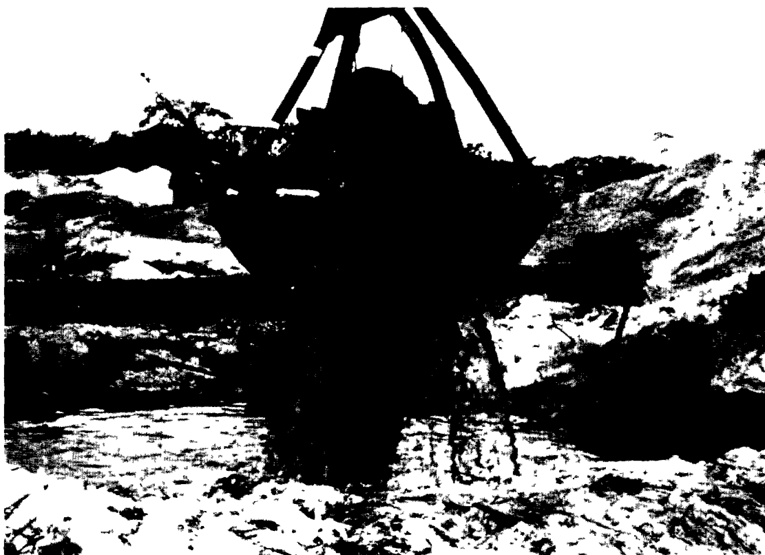
FIGURE 6-14. DEBRIS REMOVAL DURING AOMON CRYPT EXCAVATION. Long sections of "I" and "H" beams had to be removed prior to driving of sheetpile in this area. The clamshell bucket was used as a grapple to search for debris since the water in the hole was too dirty for more precise methods. (February 1979)
