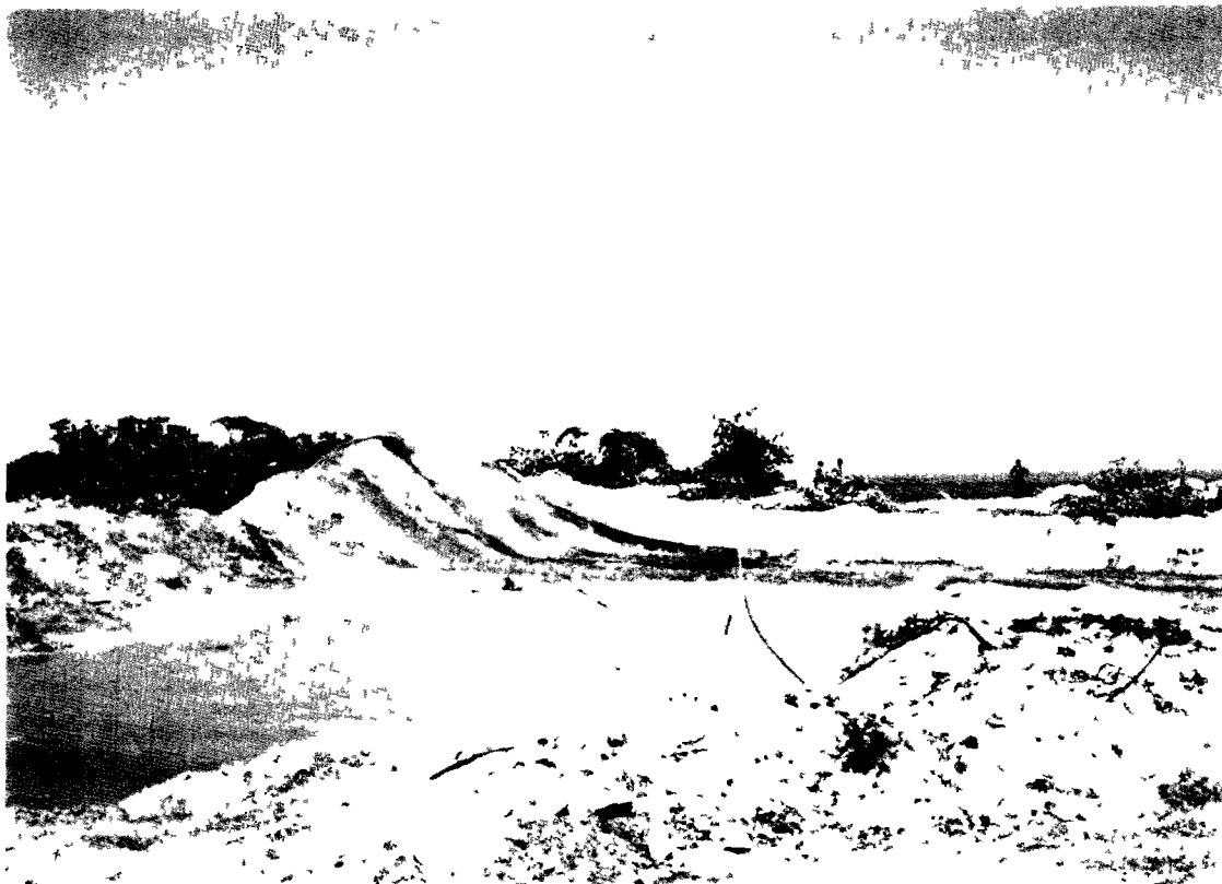
FIGURE 6-21. SUBSURFACE EXCISION ON ISLAND JANET. Soil was pushed out of the hole into a mound. The hole had standing water by the next day. Piled up soil was all removed, then the hole was backfilled and recontoured. (January 1979)
