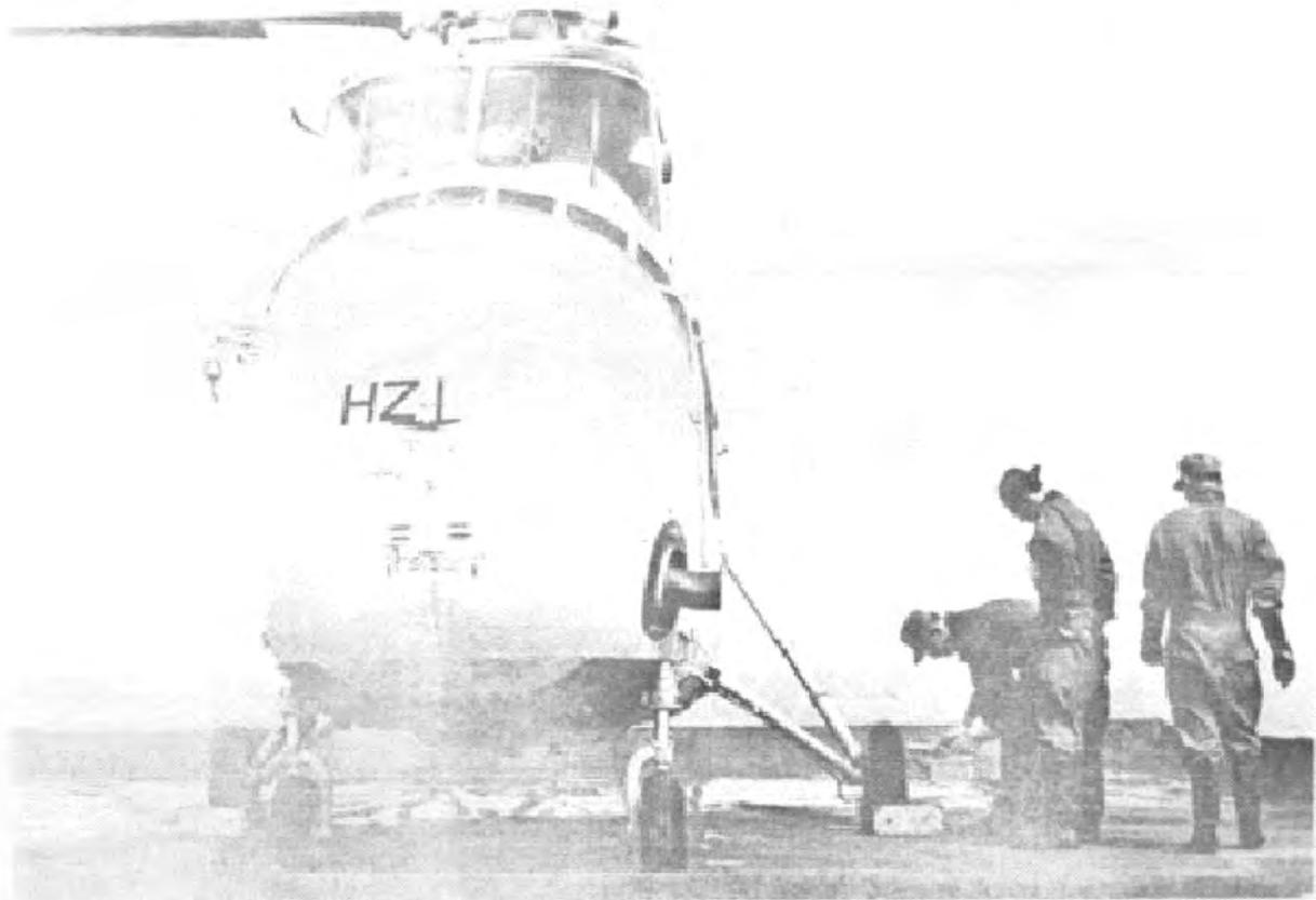
Figure 31. Helicopter in decontamination "bathtub" on USS Badoeng Strait (CVE-116), REDWING.
