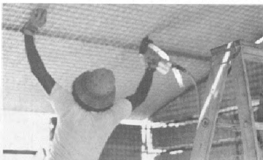
FIGURE 10-14. JOINING CEILING PANELS WITH AIR-ACTUATED CLAMPING DEVICE.
