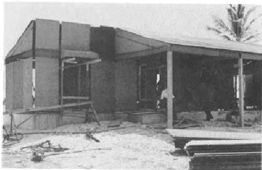
FIGURE 10-15. HOUSE NEARING COMPLETION WITH W-PANELING INSTALLED.
