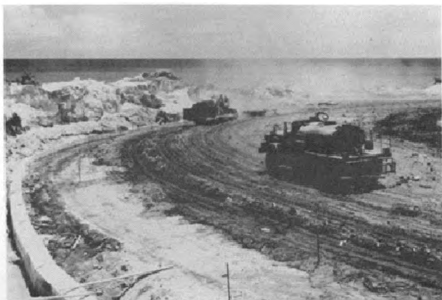
FIGURE 8-32. SPRINKLING SOIL-CEMENT MIXTURE.
