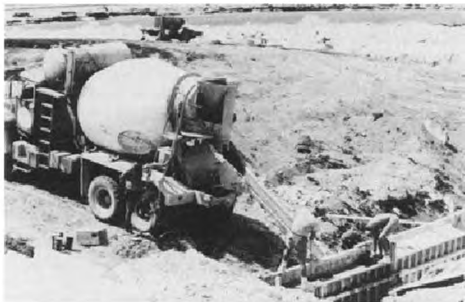
FIGURE 8-27. PLACING CEMENT IN KEYWALL FORMS.
