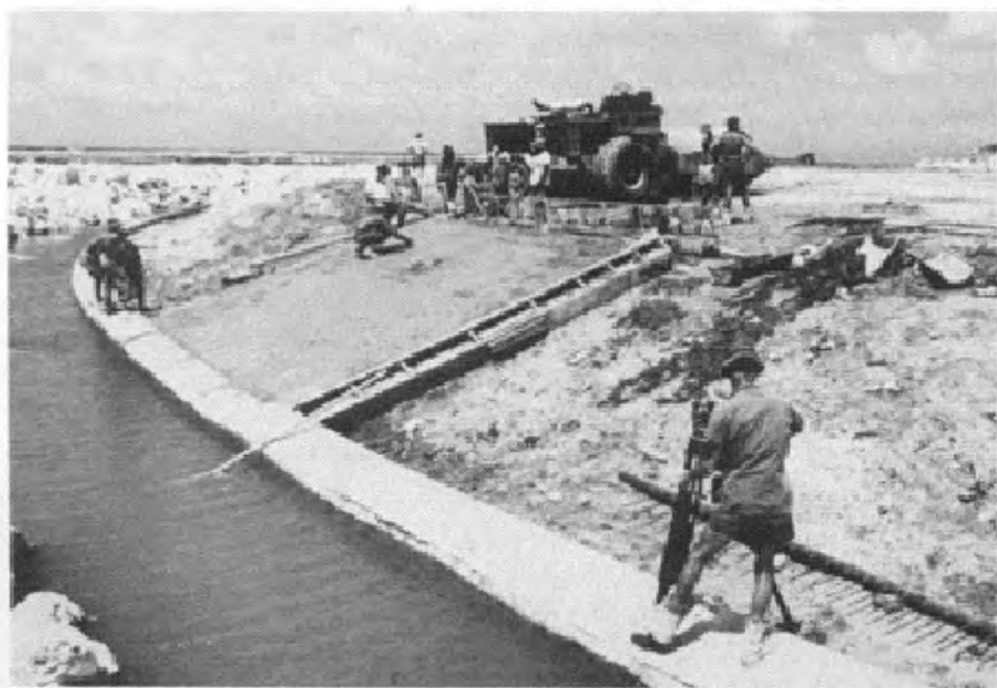
FIGURE 8-44. SIDE VIEW OF FORMS.
