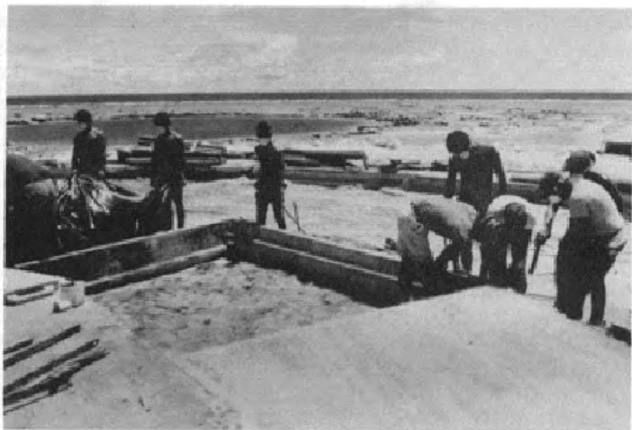
FIGURE 8-45. WOODEN CAP FORMS WITH TAPERED KEY.
