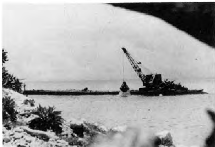
FIGURE 5-9. FLOATING PLATFORM DEBRIS REMOVAL.
