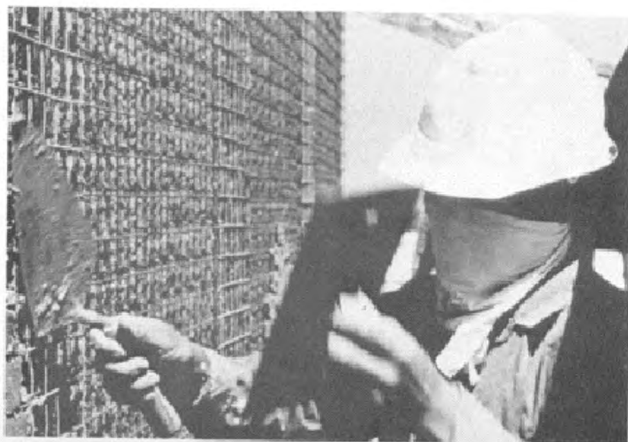
FIGURE 10-16. APPLYING CEMENT PLASTER.
