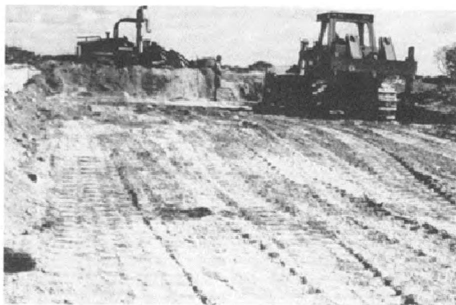
FIGURE 6-6. BACKBLADING OPERATION.
