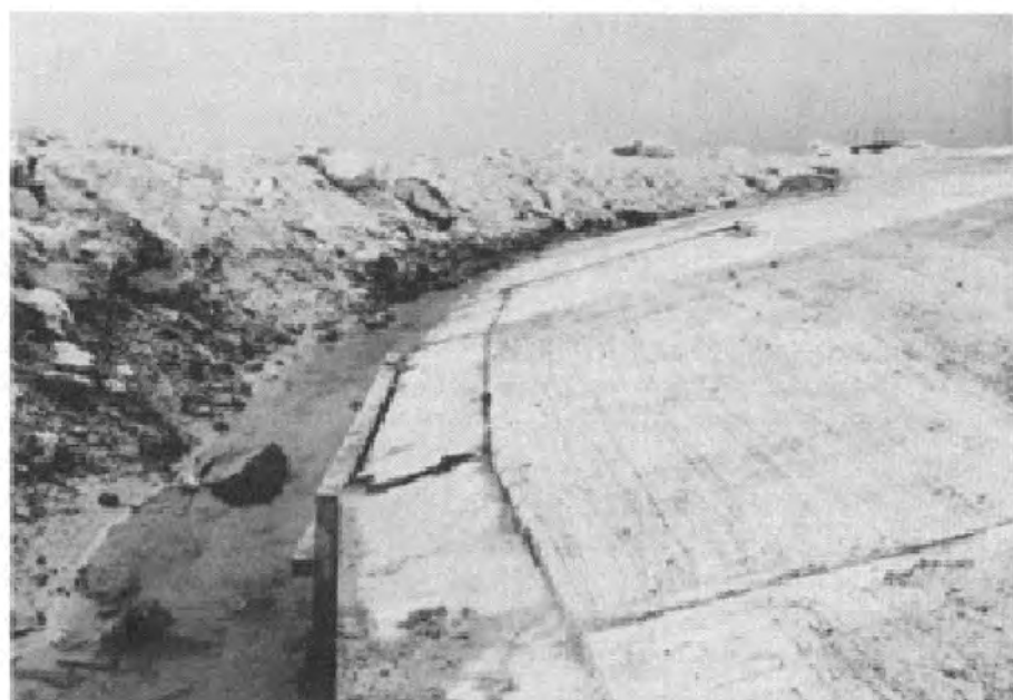
FIGURE 8-43. KEYWALL EXPANSION JOINT.
