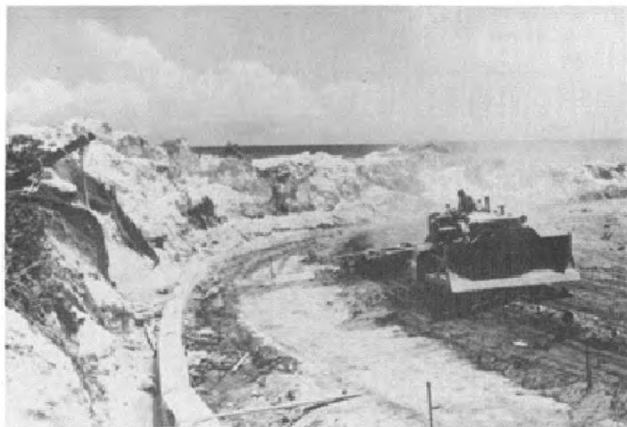
FIGURE 8-31. MIXING SOIL AND CEMENT WITH DISC HARROW.
