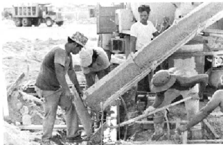
FIGURE 10-12. PLACING CONCRETE FOR HOUSE FOOTINGS.
