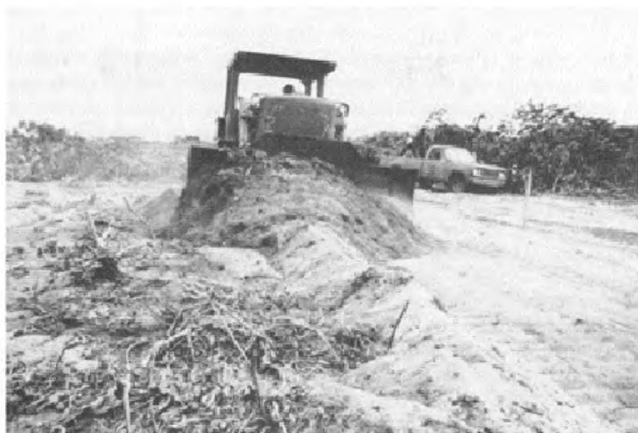
FIGURE 6-4. SOIL REMOVAL USING D8K DOZER.
