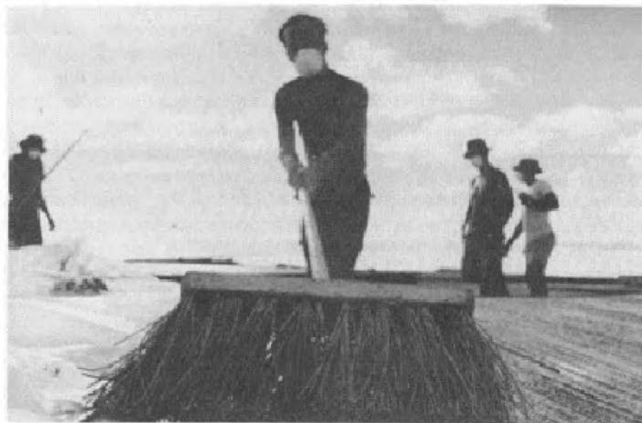
FIGURE 8-48. BROOM-FINISHING A CAP SECTION.
