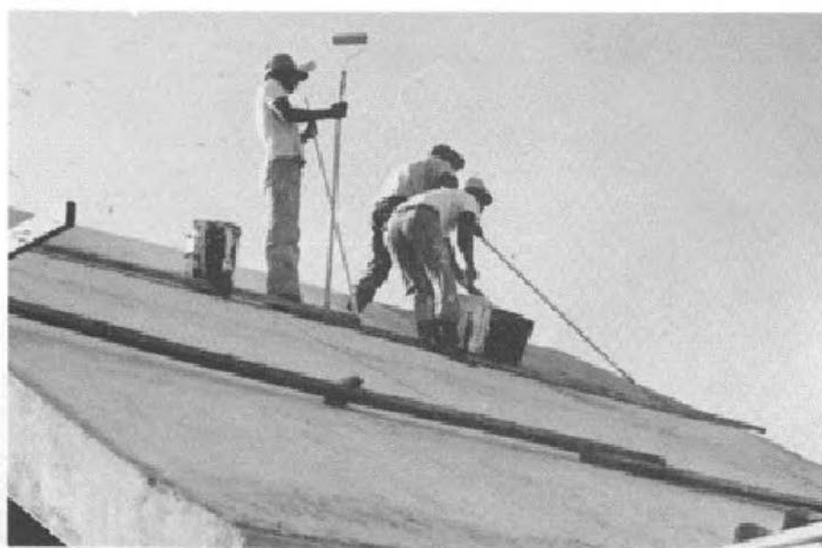
FIGURE 10-18. PAINTING THE ROOF.
