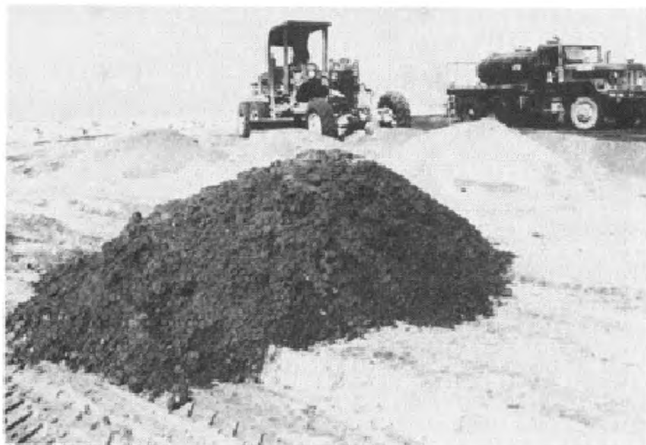
FIGURE 8-29. SPREADING SOIL WITH A GRADER.
