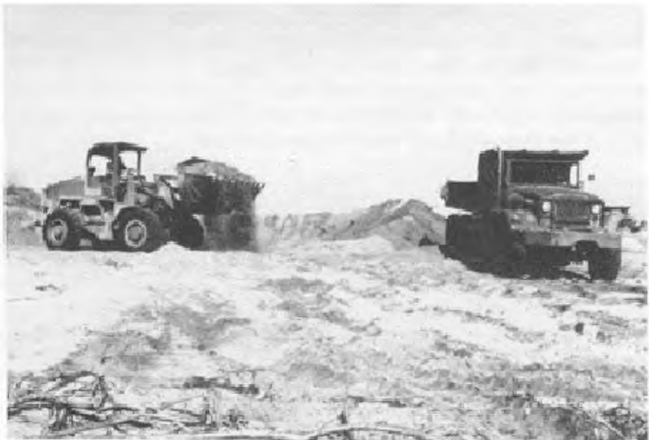
FIGURE 6-9. CONTAMINATED SOIL MOVEMENT.
