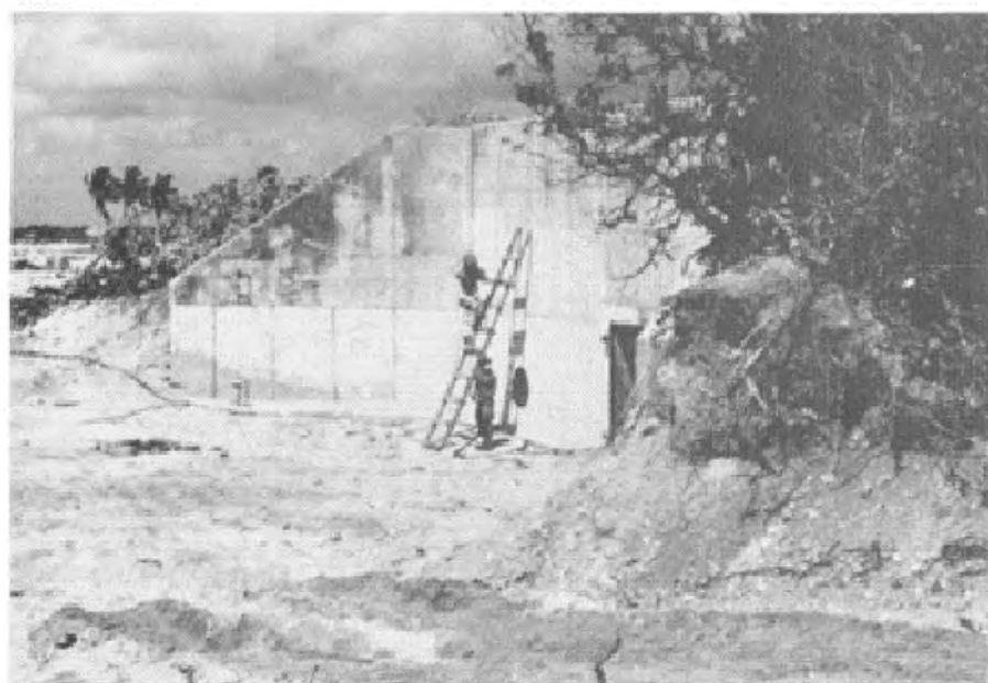
FIGURE 5-25. BUNKER SAND-BLASTING OPERATION.
