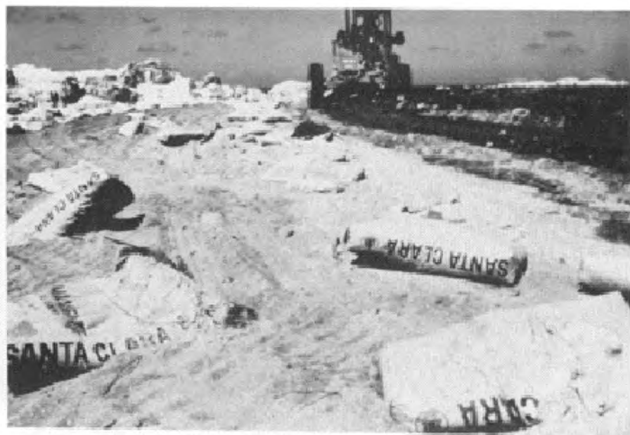
FIGURE 8-30. CEMENT BAGS PLACED FOR SOIL-CEMENT MIX.
