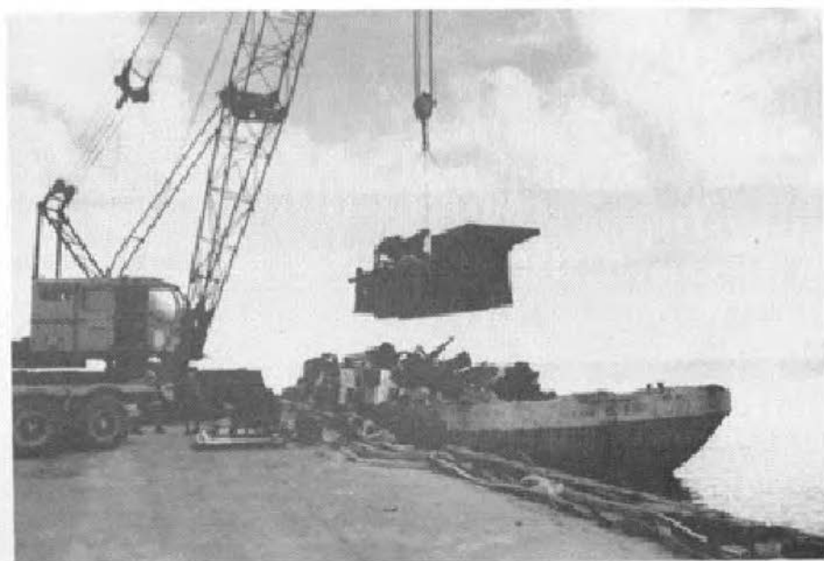
FIGURE 5-16. DUMP BED OFFLOADING.
