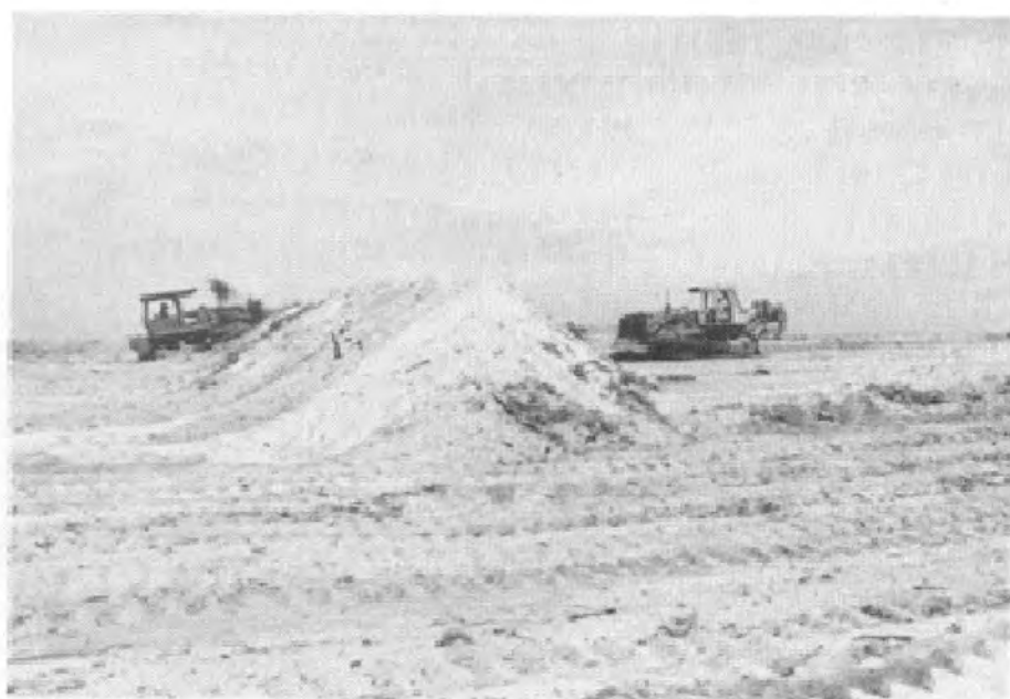
FIGURE 6-7. SOIL WINDROWING.
