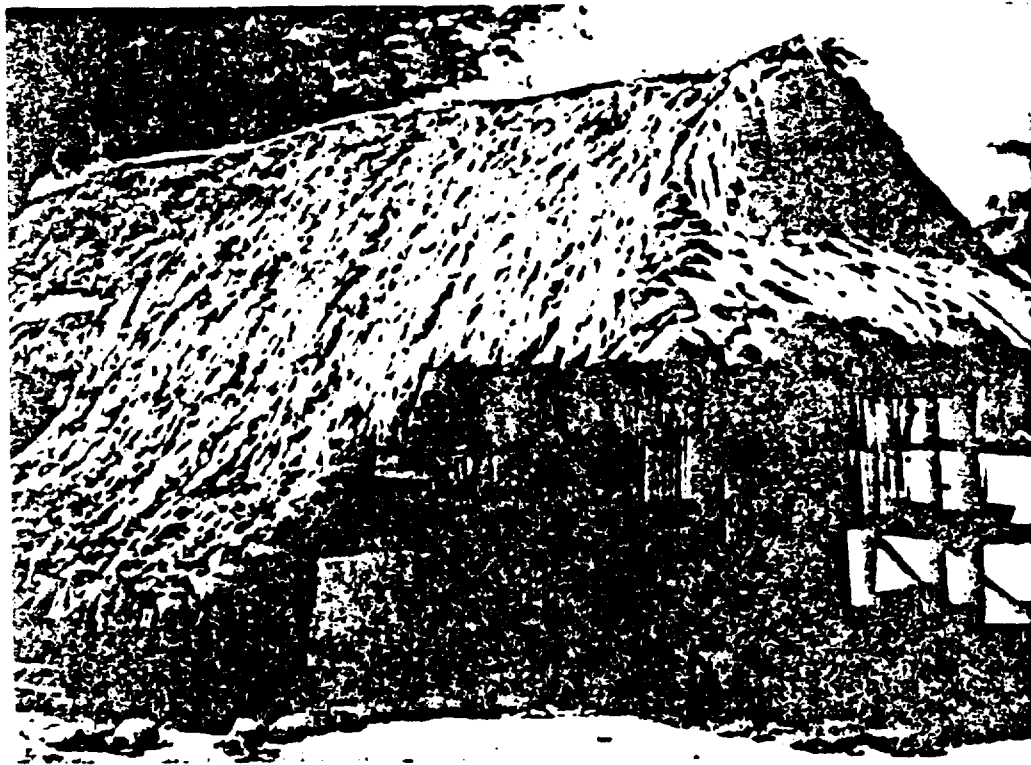
Figure 2.5 Typical dwelling, illustrating open-type construction, lean-to roof, and an area for preparing meals "indoors" during rainy weather.
