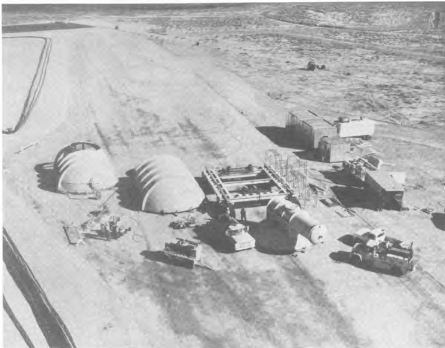
Figure 7.2 HURON KING event - major components of the experiment tank prior to assembly.
