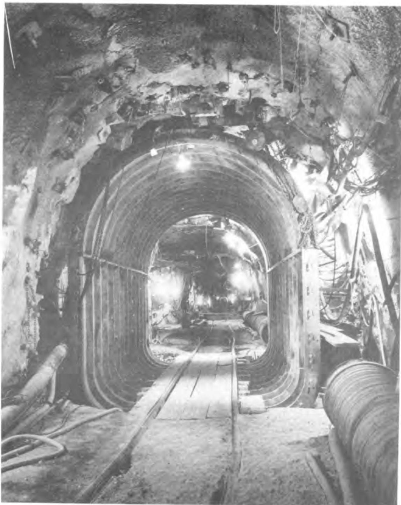
Figure 8.2 MINERS IRON event - OBP before concrete pour.
