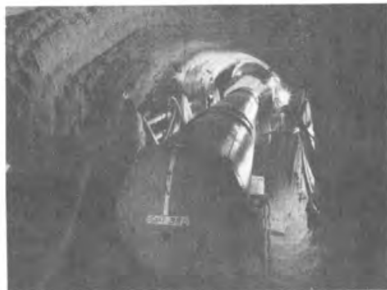
Aggebian water tank in E drift after partial stemming pour
