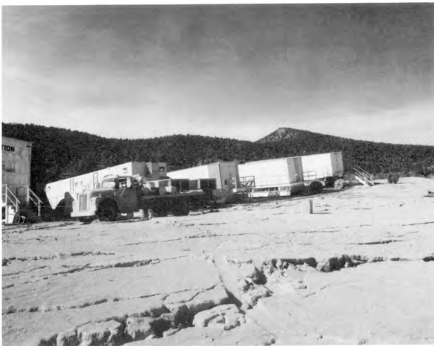
Figure 6-9. MIDAS MYTH/MILAGRO event - mesa trailer park subsidence damage.
