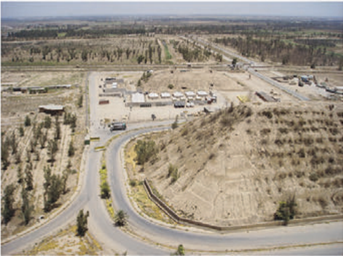
Bunker B at Tuwaitha Nuclear Research Center, Iraq
