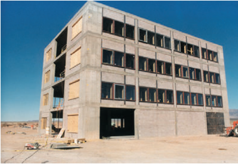
At Albuquerque, DTRA used the Divine Buffalo test series to measure the blast effects of high explosive weapons on redesigned building structures.
