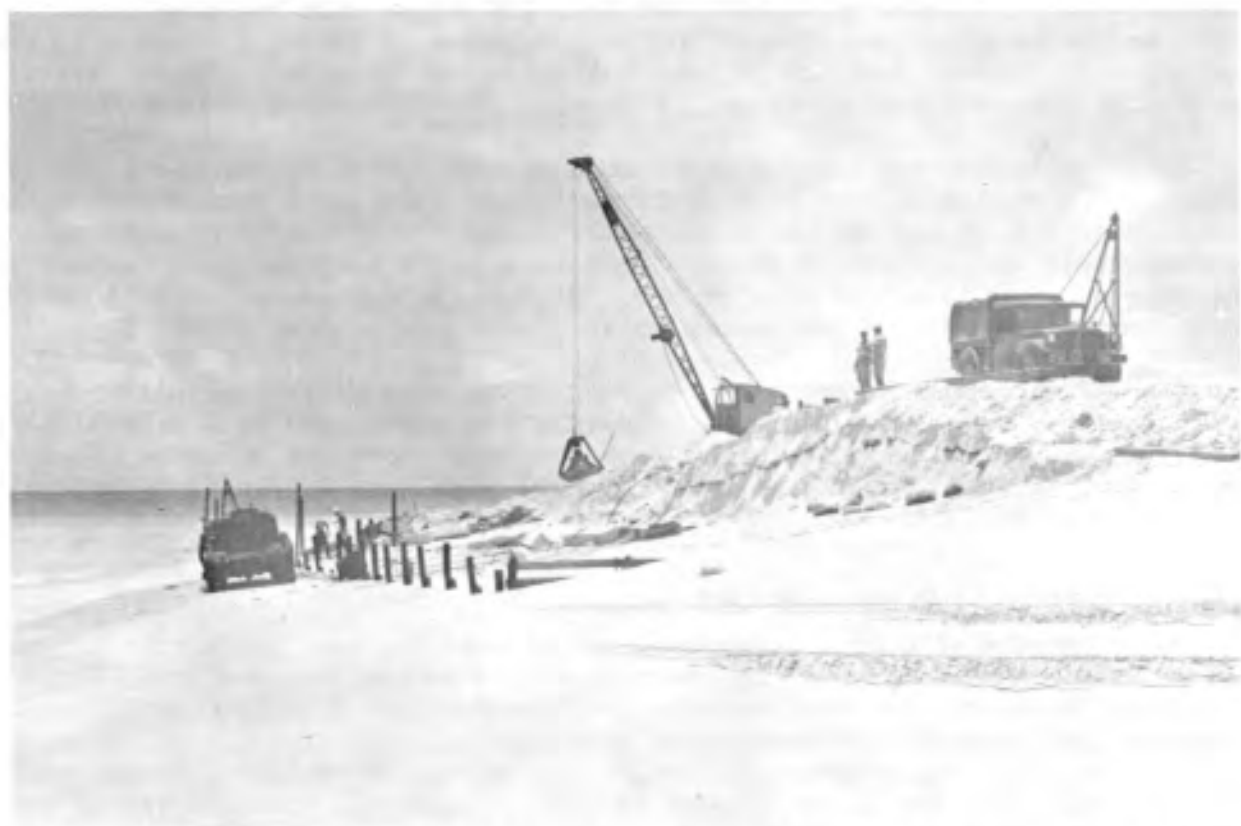
Figure 12. Revetment being built at west end of Eneman Island, Bikini Atoll (tip of ZUNI crater), 1958.
