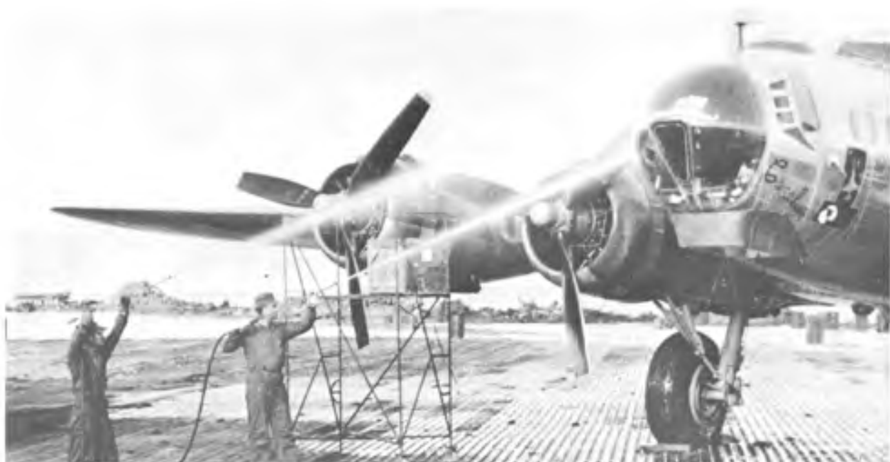
Figure 35. Decontamination of SANDSTONE B-17 drone sampler.
