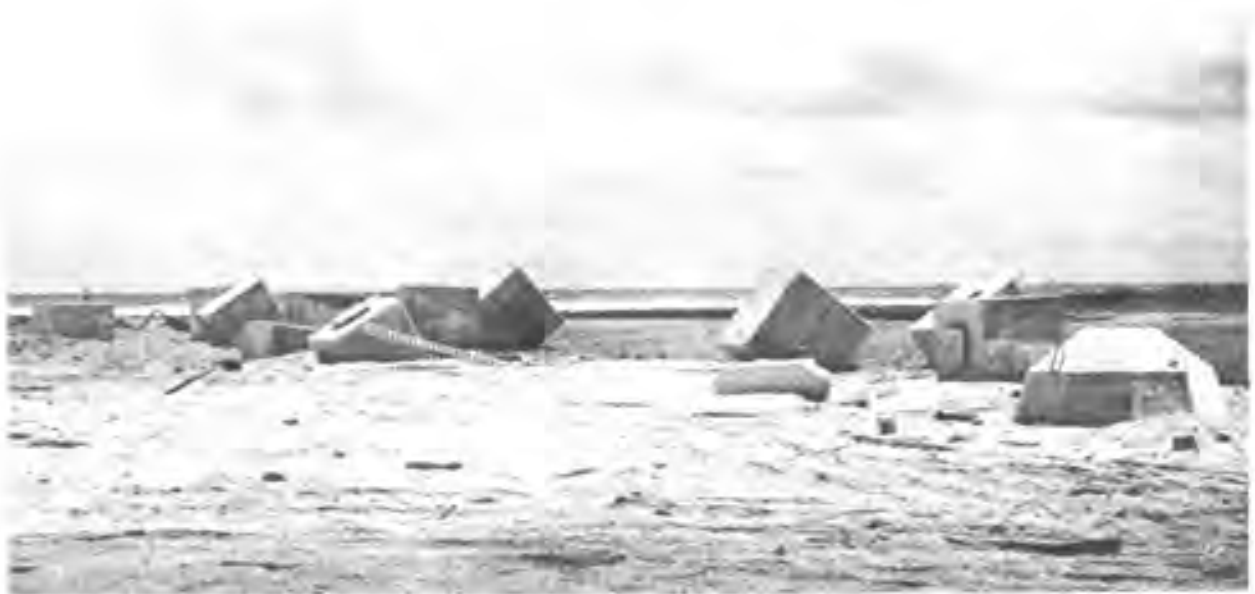
Figure 41. Navy Bureau of Yards & Docks experimental structural shapes after shot YOKE, Operation SANDSTONE.
