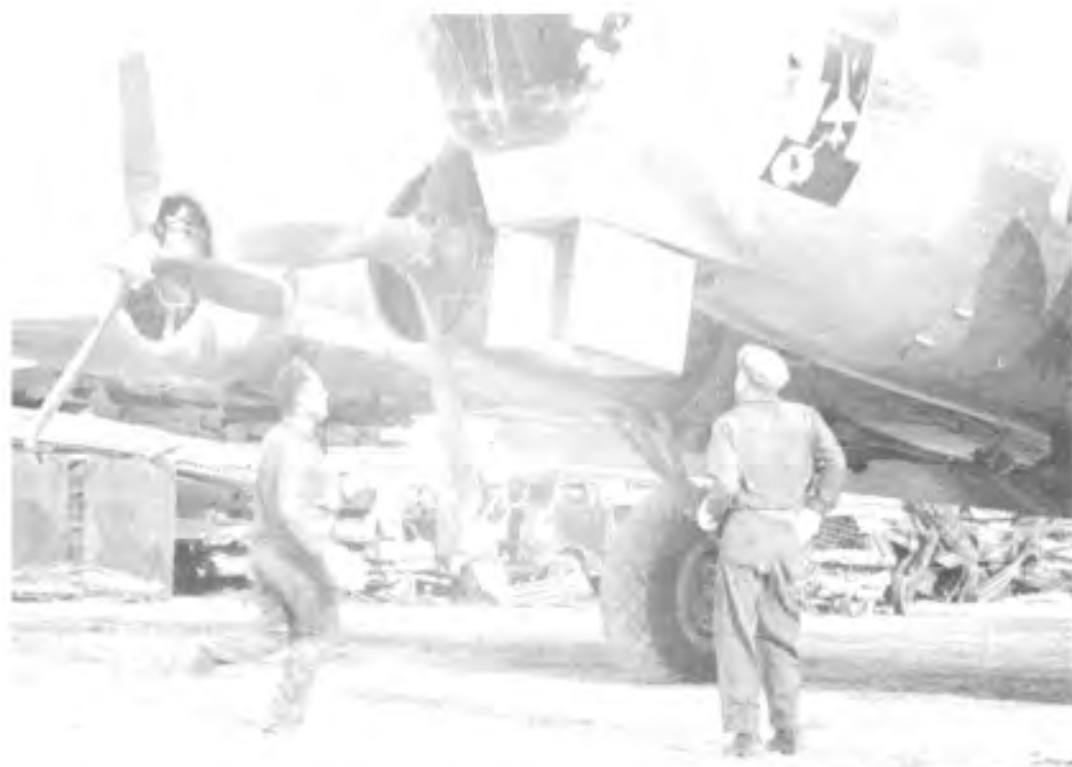
Figure 24. Two men run in to pull filter holders from lower sampler on B-17 drone following shot ZEBRA, Operation SANDSTONE. Junk revetment is in background.
