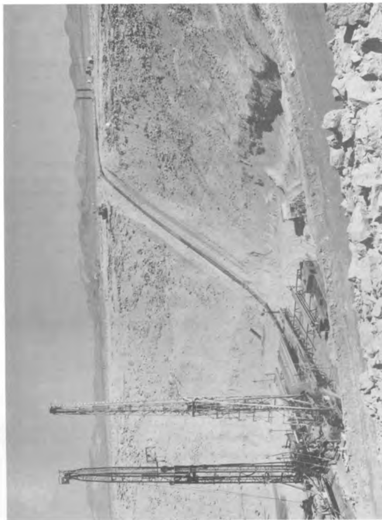
Figure 2.1 A Typical Subsidence Crater and Postevent Drilling Operation
