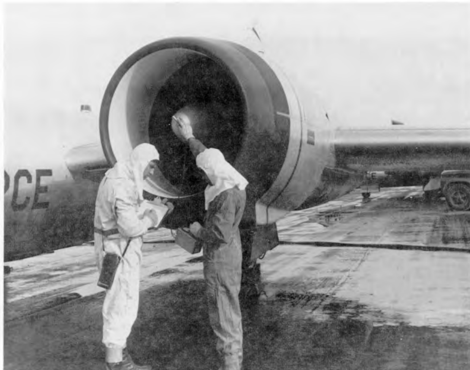
Figure 2.8 Air Force and Radsafe personnel monitoring a B-57 after decontamination.
