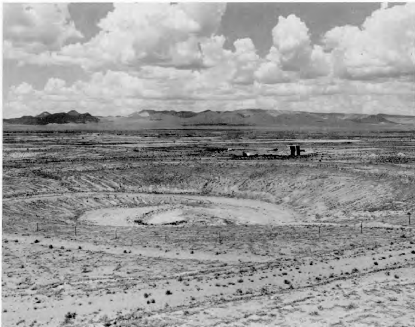
Figure 2.1 A typical subsidence crater.
