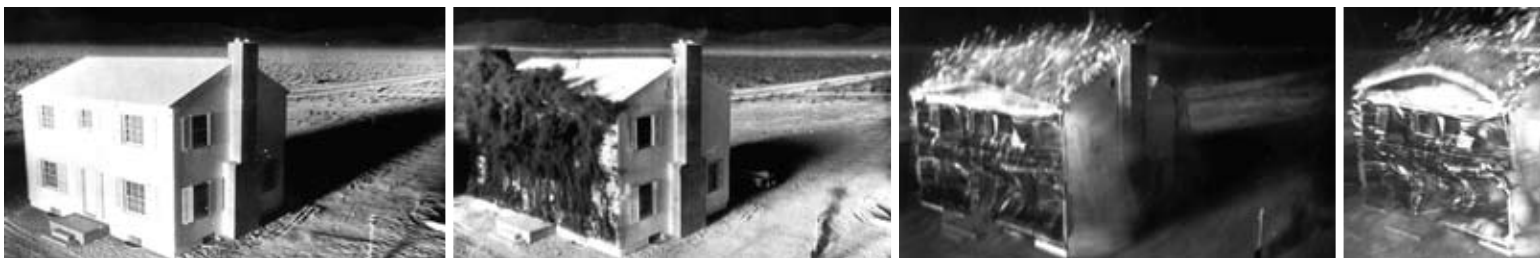
Complete destruction of House No. 1 , located 3,500 feet from ground zero, by an atomic blast at Yucca Flat at the Nevada Proving Ground – March 17, 1953.
